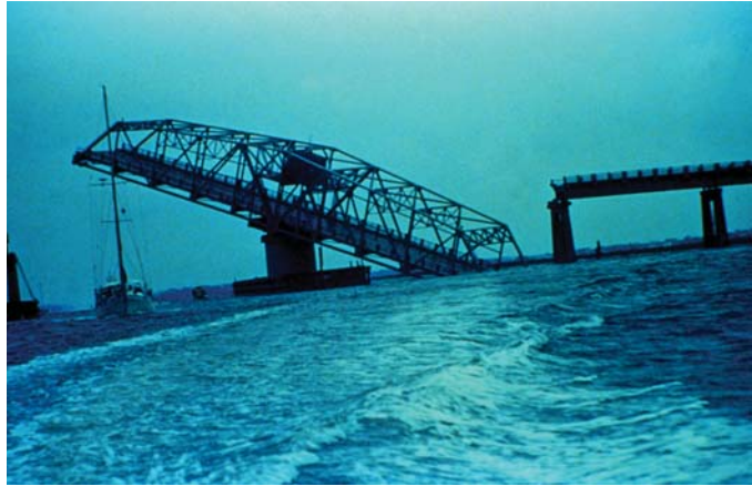
Hurricanes have the capacity to destroy critical infrastructure. Depicted here, Hurricane Hugo obliterated Ben Sawyer Bridge to Sullivan's Island, SC.
